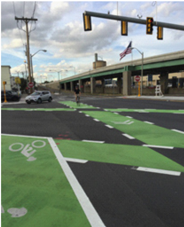
New markings at the Somerville Ave/Medford St intersection
